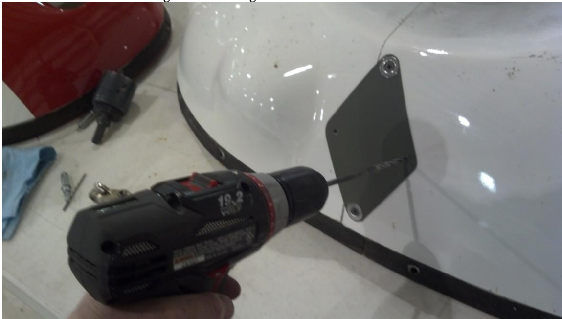
Figure 7 - Mount AC-00942 cover and match drill
