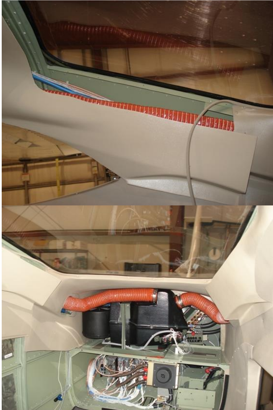
Figure 12 - SCAT Tubing Installation
