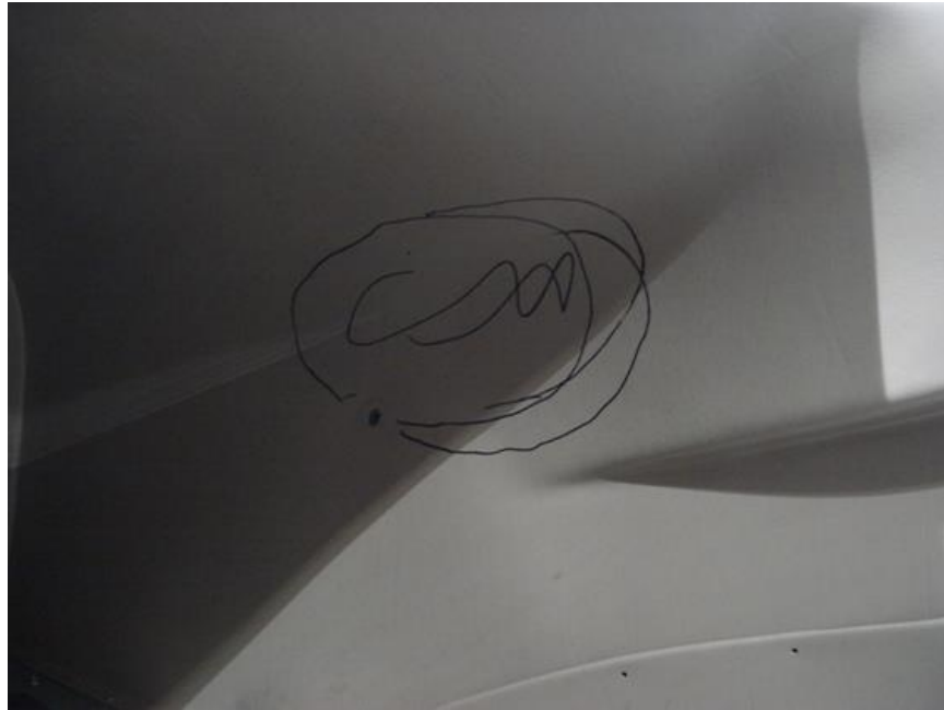
Pilot Side looking at baggage compartment panel assembly
