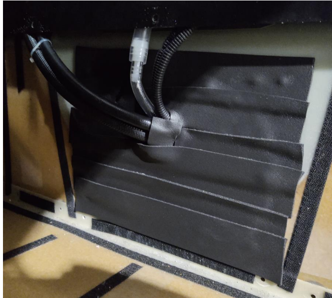
Figure 8 – Seal with Foam
