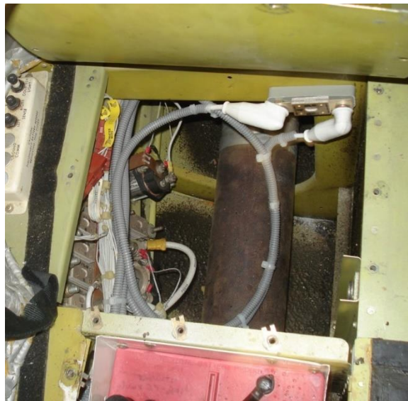
Figure 21 – Baron 58 Current Limiter Installation
