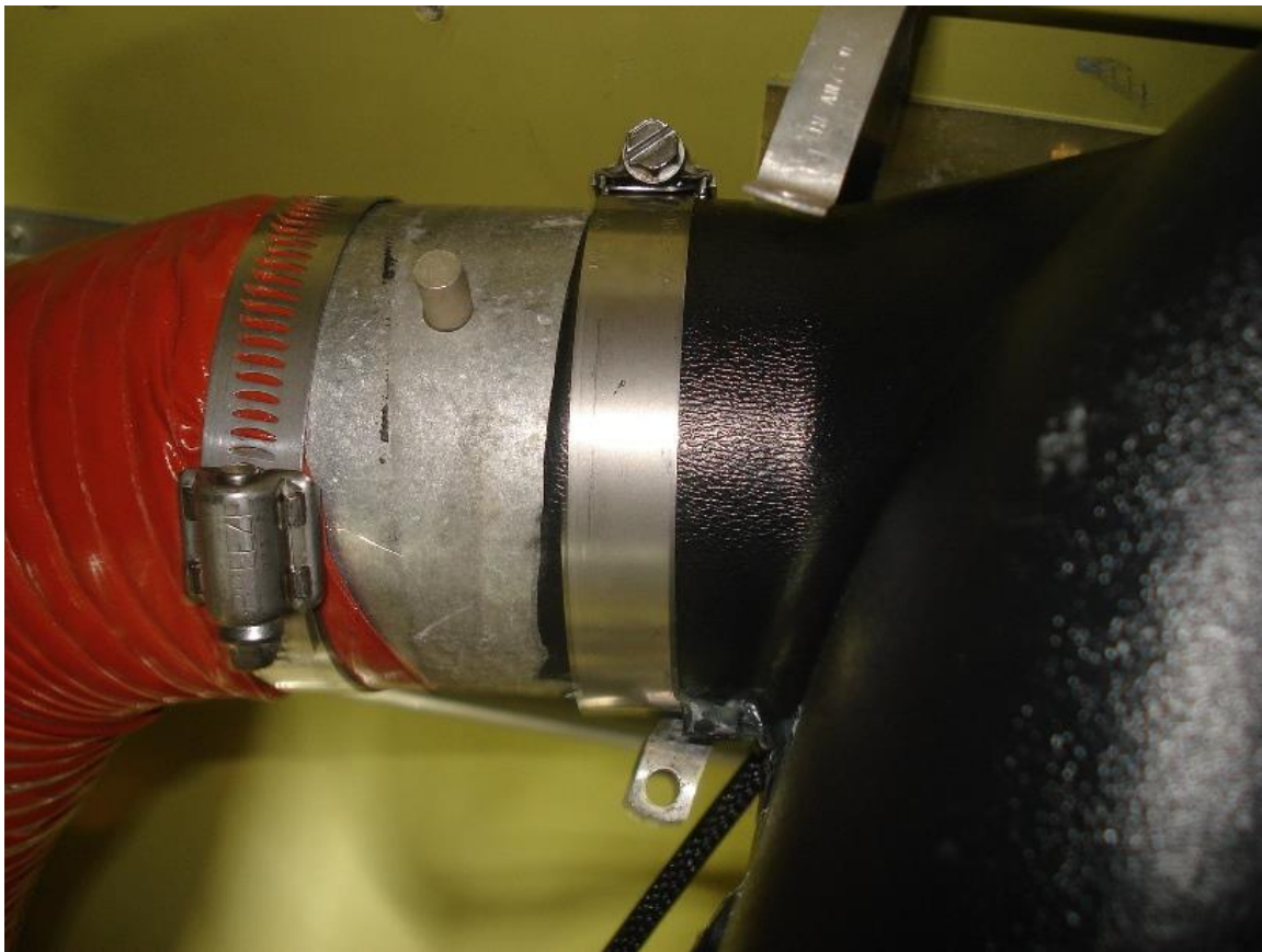
Figure 12 - Shutoff Valve and Tubing Install
