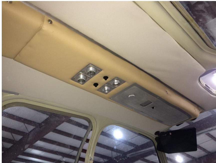
Figure 9 - Install Forward Duct Cover Assembly
