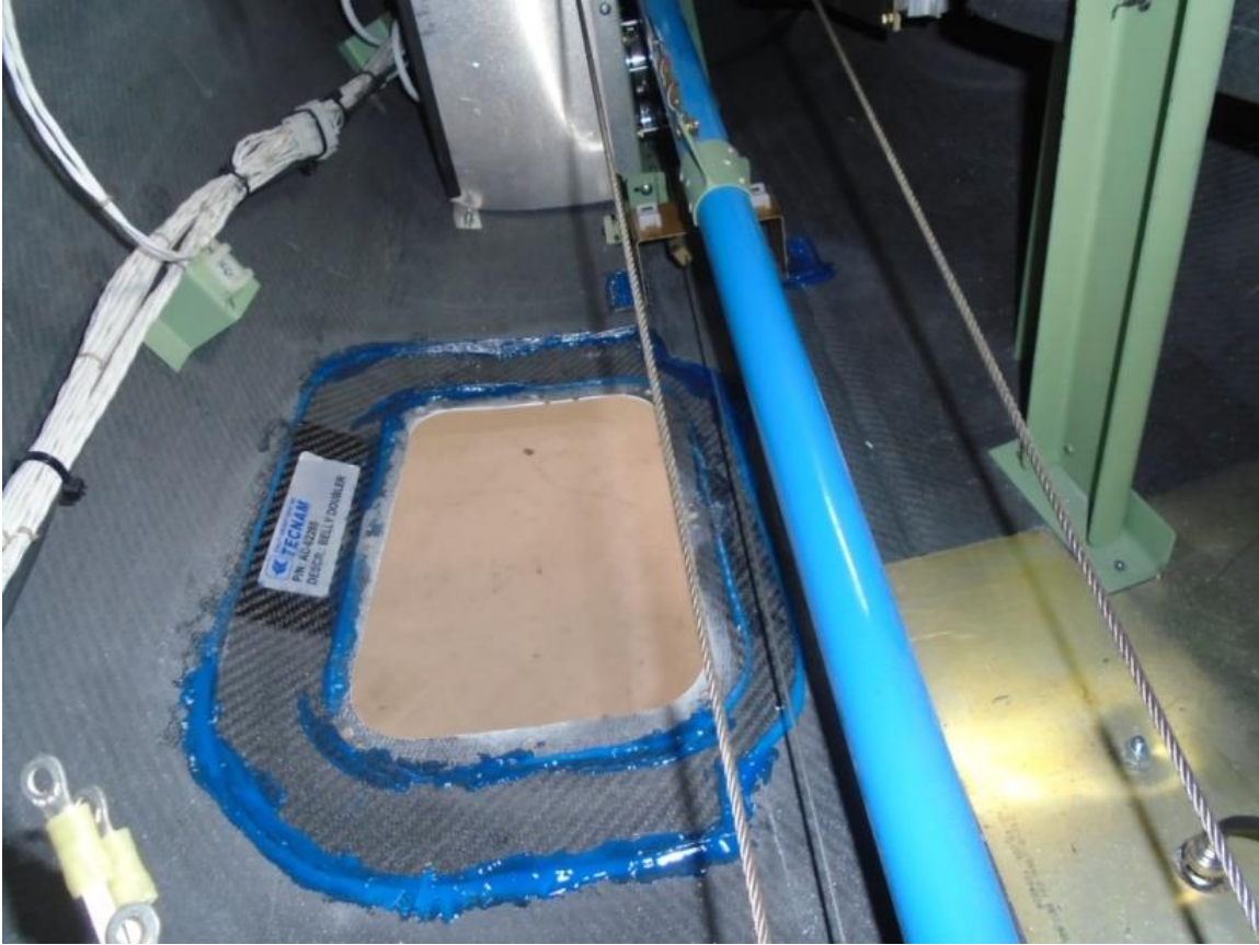
Figure 1 – Belly Doubler Installation
